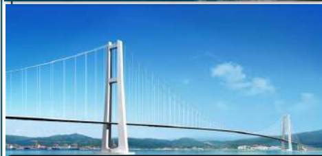
Gwangyang Long-Span Bridge
