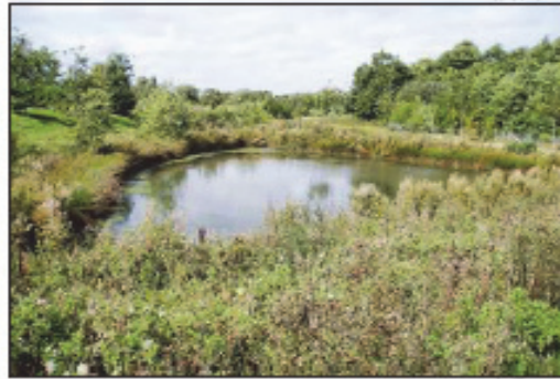
Typical Attenuation Wet Pond
