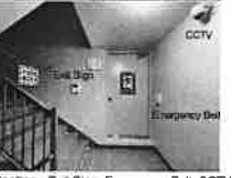
Rooftop : Exit Sign, Emergency Bell, CCTV
